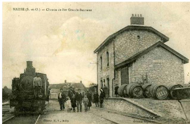
Station de Maisse
